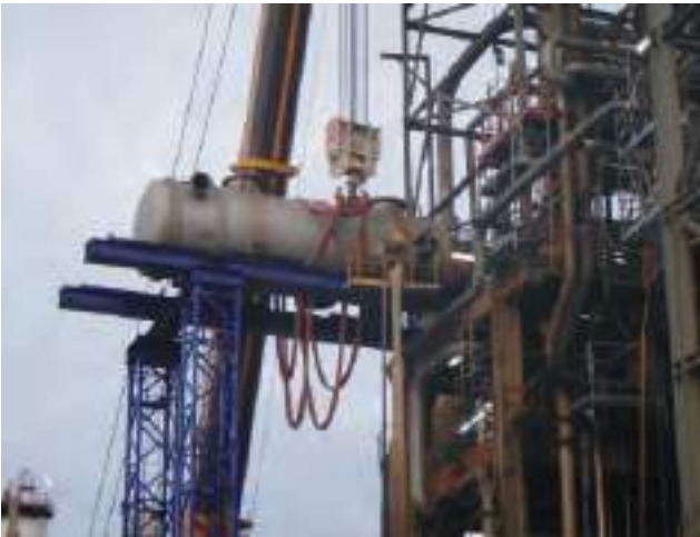
Heat exchanger replacement
