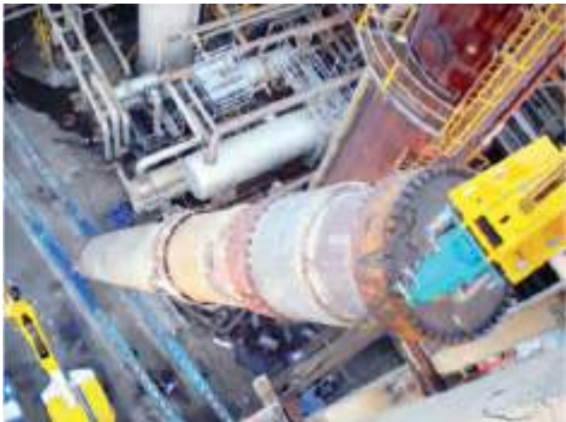
Extraction and insertion of Exchanger
