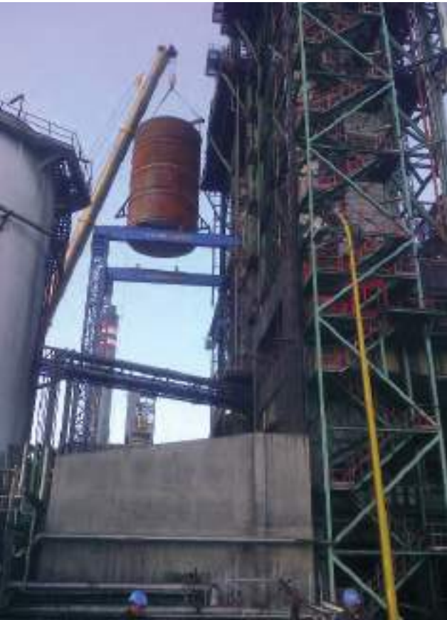
Section replacement of the coke drums.
