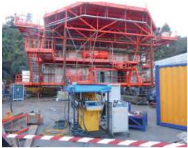
Weighing of modules of regasification platform
