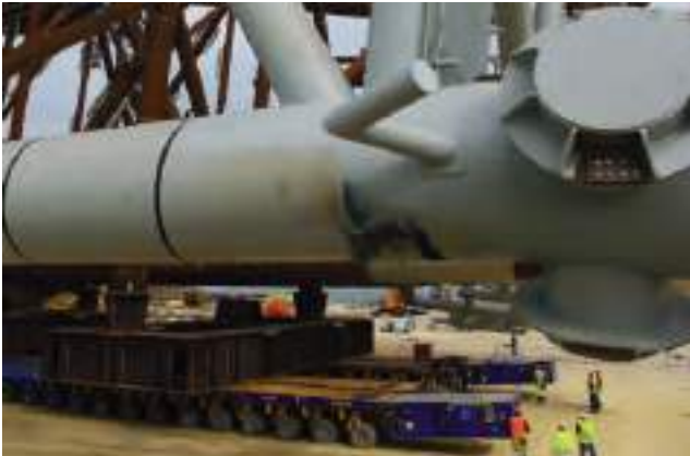
Weighing, Ballasting and load out: Puq Jacket of 4.480,6 Tn.
